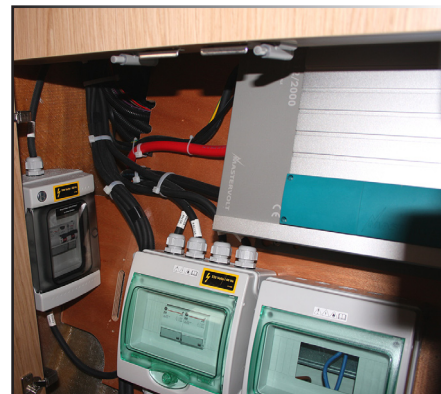
CONSUMING APPLIANCES CIRCUIT BREAKERS
